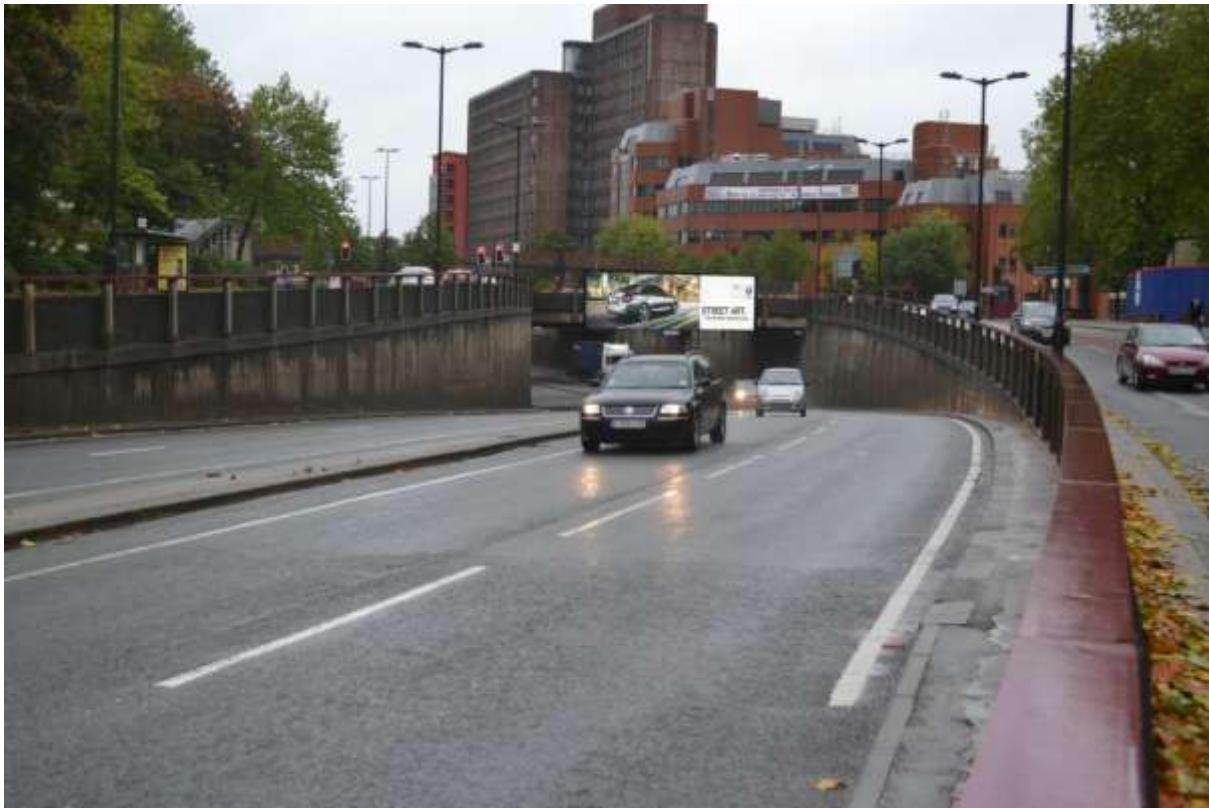
Old Market Roundabout Underpass - Northbound
