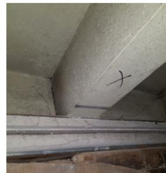
PHOTO OF TYPICAL -120 x 220 JOIST END TO BE REMEDIATED
