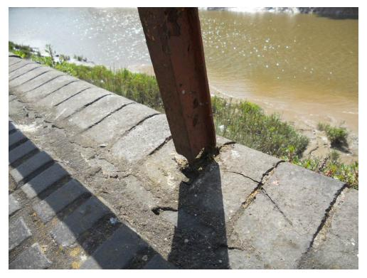
Photo 12 – Localised Severe Corrosion to Base of Parapet Post (Ch140m)
