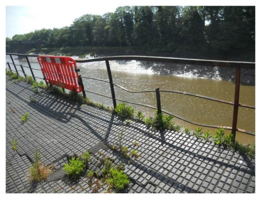
Photo 10- Major Distortion of Railings at Centre of Slip (Ch170m)
