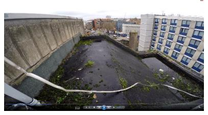
**Figure 5-4 Main stairwell roof**Deterioration of roofing material, standing water and detachment of lightning strip from file GOPR0427
