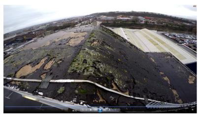
**Figure 5-6 Southwest corner stairwell roof** *Roofing material in degraded condition, and lightning strip from file GOPR0429*
