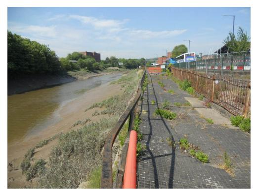
Photo 11 – Major Distortion of Railings at Centre of Slip (Ch170m)
