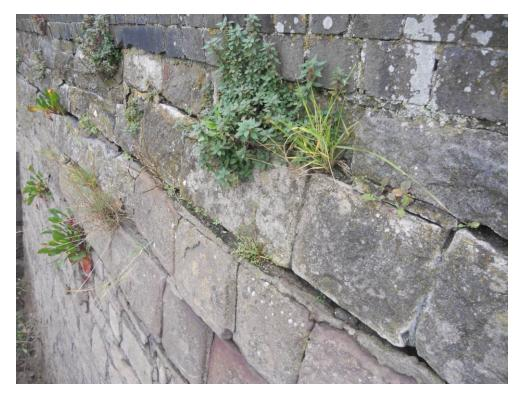
Photo 07 - Displaced Stonework Between Buttress B13 and B14 (Ch157m - 160m)
