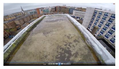
**Figure 5-5 Lift motor room roof**Roofing material in good condition, standing water and lightning strip from file GOPR0428
