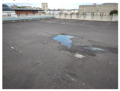
Figure 5-7. Northeast corner of the car park, Level 7B Worn area of bituminous surfacing material
