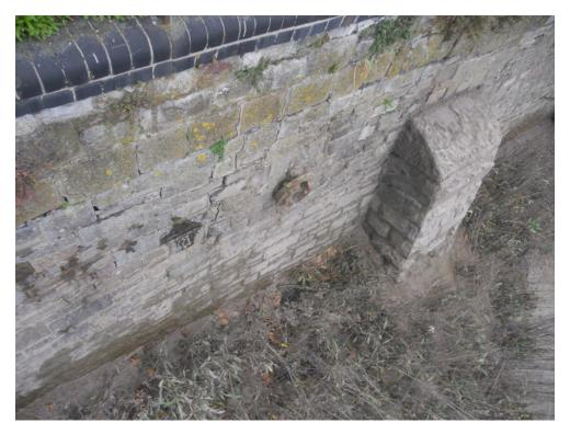
Photo 05 - Cracks in Wall Near to Buttress B11 (Ch144m)
