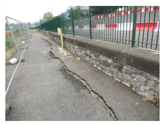
Photo 21 – Tension Crack in Tarmac over Railway (Ch147m – 195m)
