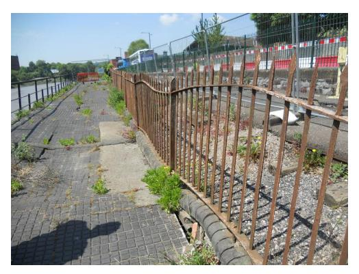
Photo 23 – Major Deformation of Railway Railings Due to Ground Movement (Ch165m)
