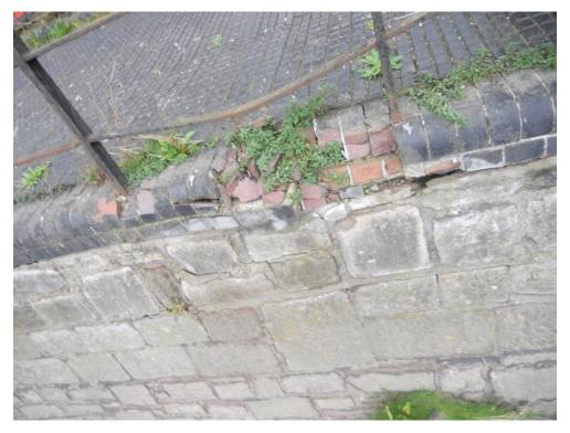
Photo 08 – Displaced Brickwork Above Buttress B15 (Ch168m)
