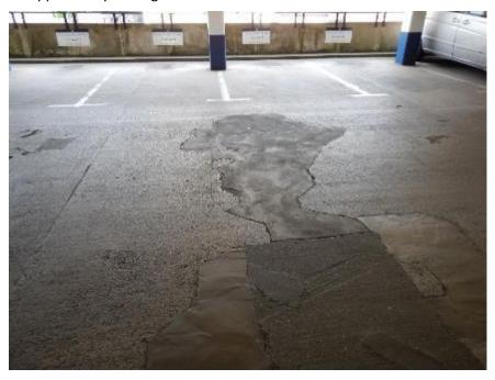
Figure 5-5. Spalling to lower level deck Multiple phases of repair to the deck in the turning area over an extensive area
