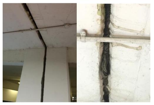
Figure 5-9a (left) and 9b (right). Expansion joint at columns and soffit, intermediate level Note mastic-like sealant between the columns and rope-like infill to the soffit joint.
