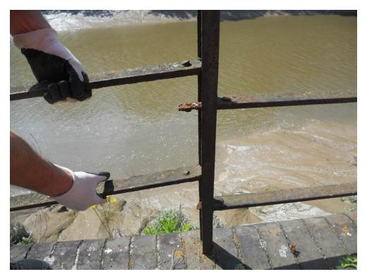
Photo 13 – Corroded Fixings to Intermediate Rails (Ch210m)
