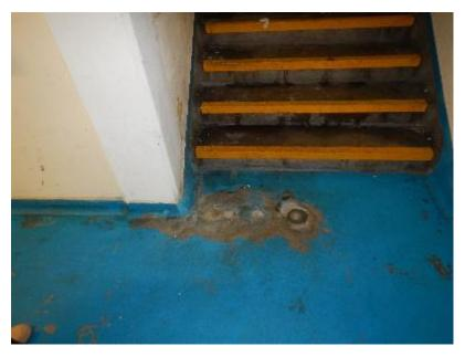
Figure 5-10. Main stairs at Level 6A Note painted floor, anti-slip nosings to the treads and stalagmites forming below leaking concrete roof.
