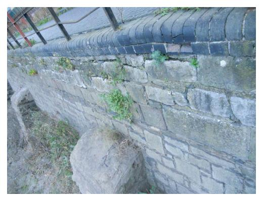
Photo 09 - Mortar Deterioration above Buttress B17 (Ch180m)
