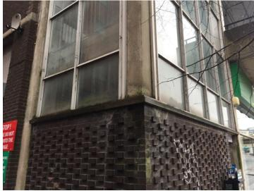
Figure 5-15 External views of stairwell Views illustrating façade glazing, stair units, structural frame and brickwork
