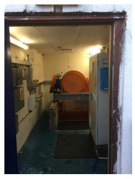
**Figure 5-7 Lift motor room**Room in good condition with no obvious sources of water ingress
