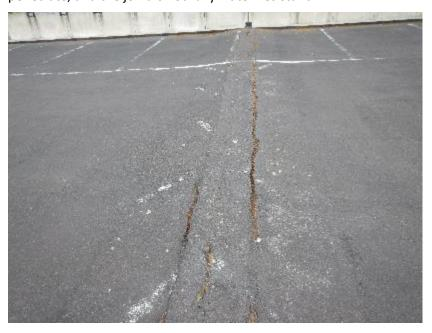
Figure 5-8. Roof-level (7B) expansion joint
