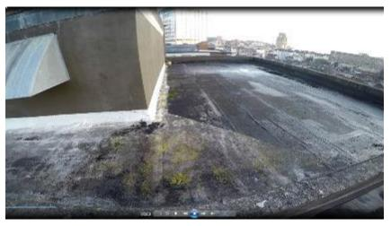
**Figure 5-12 Main stairwell roof** *Roofing material in good condition and standing water from file GOPR0423*
