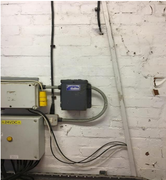
Figure 47: Unsupported cables
