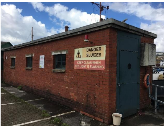
Figure 39: Emergency sluices building
