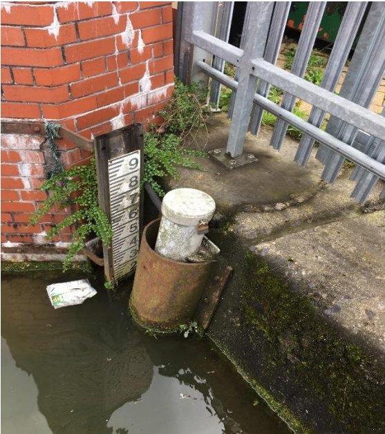
Figure 26: Harbour's level measuring instrument
