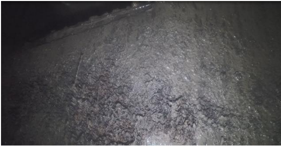
Figure 14: Condition of gate – main sluice gate 3
