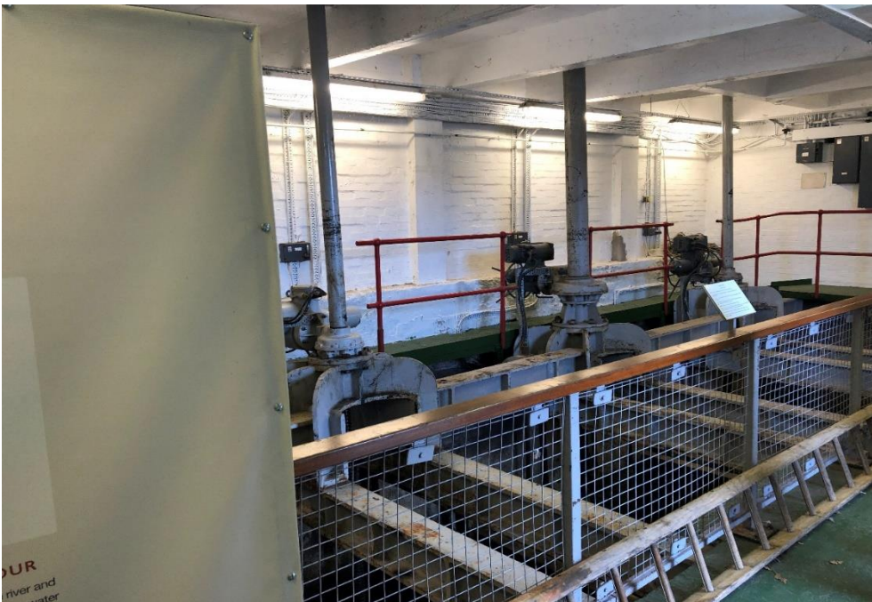
Figure 3: Underfall Yard Main Sluice Room
