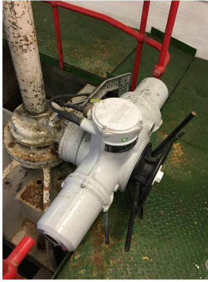
Figure 37: Actuator No.1 with cable glands
