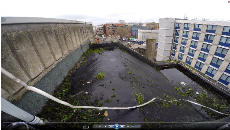
Figure 5-4 Main stairwell roof
