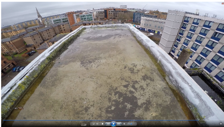
Figure 5-5 Lift motor room roof
