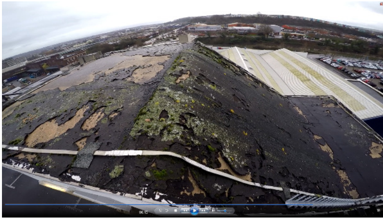
Figure 5-6 Southwest corner stairwell roof
