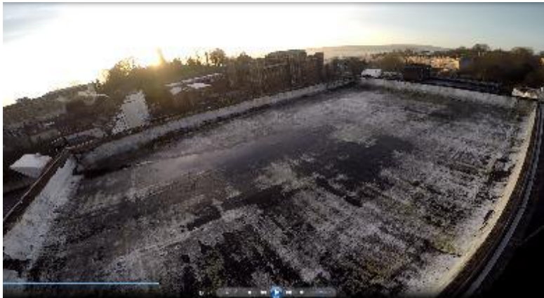
Figure 5-11 Lift motor room roof
