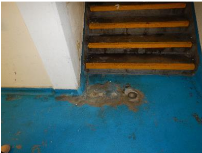
Figure 5-10. Main stairs at Level 6A
