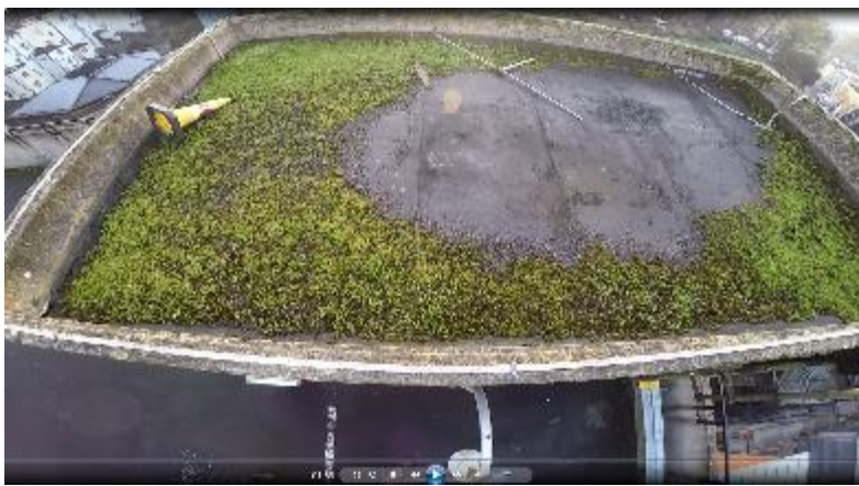
Figure 5-16 South corner stairwell roof
