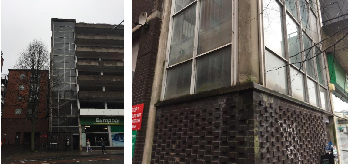
Figure 5-15 External views of stairwell
