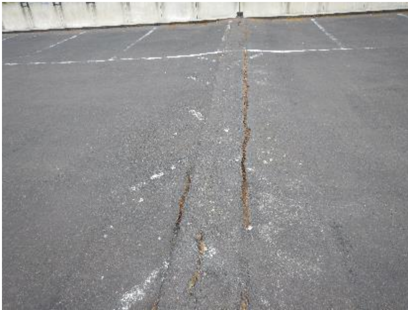
Figure 5-8. Roof-level (7B) expansion joint
