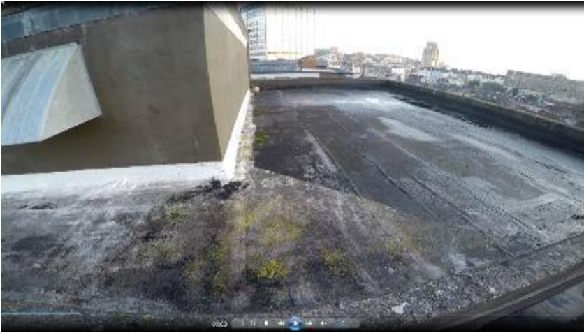
Figure 5-12 Main stairwell roof
