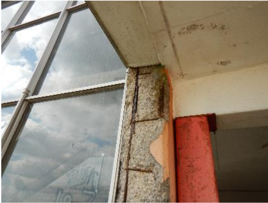
Figure 5-2. Column at south corner of car park, Level 6B
