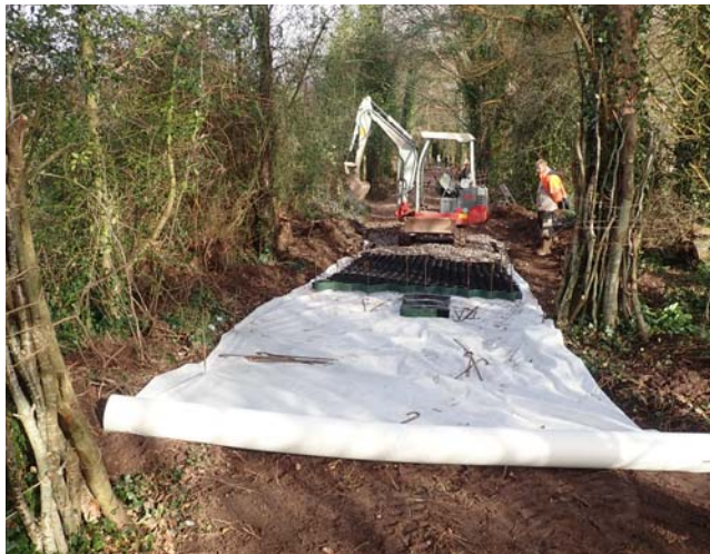
Below and right: construction of Ashton Park Link, Greenways & Cyclerroutes 2020
