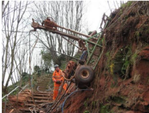
Figure 4 - Example drilling rig
