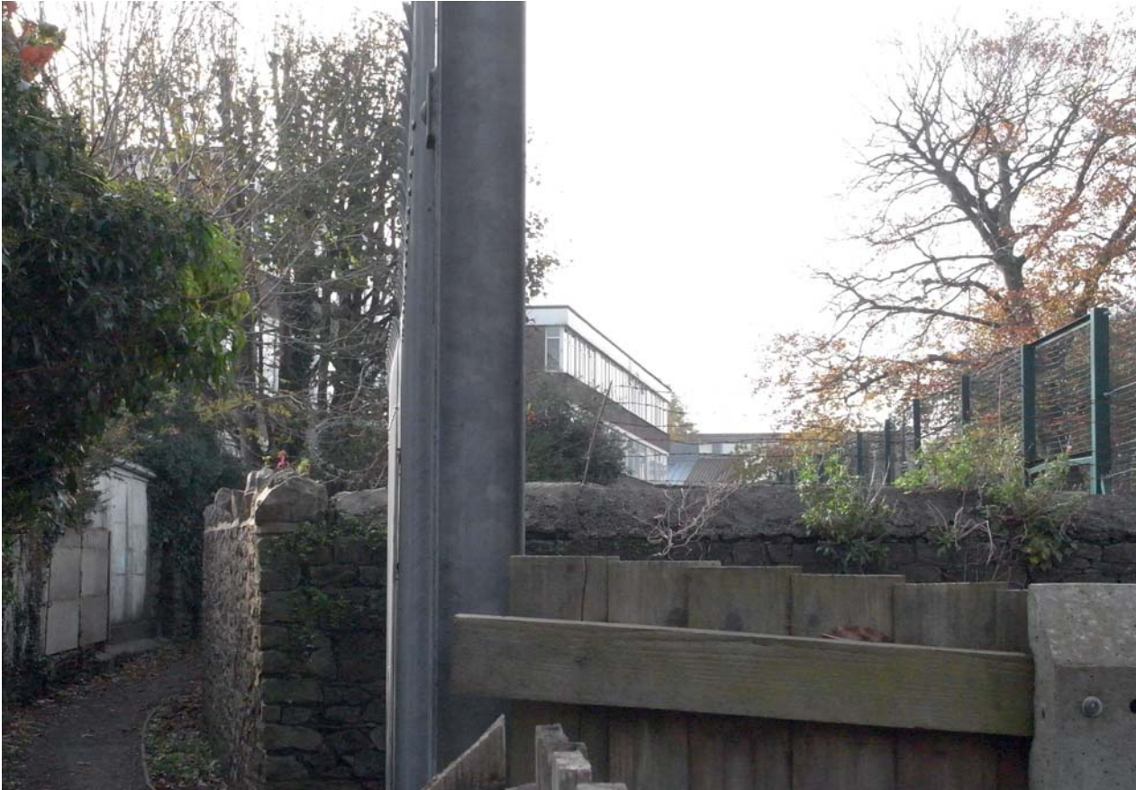
BEFORE - 3 LEVELS - Rear of building
