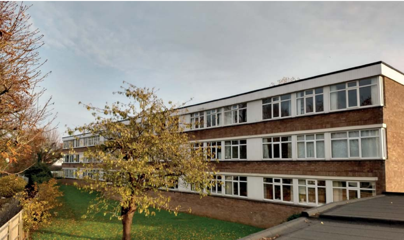
BEFORE - 3 LEVELS - Rear of building
