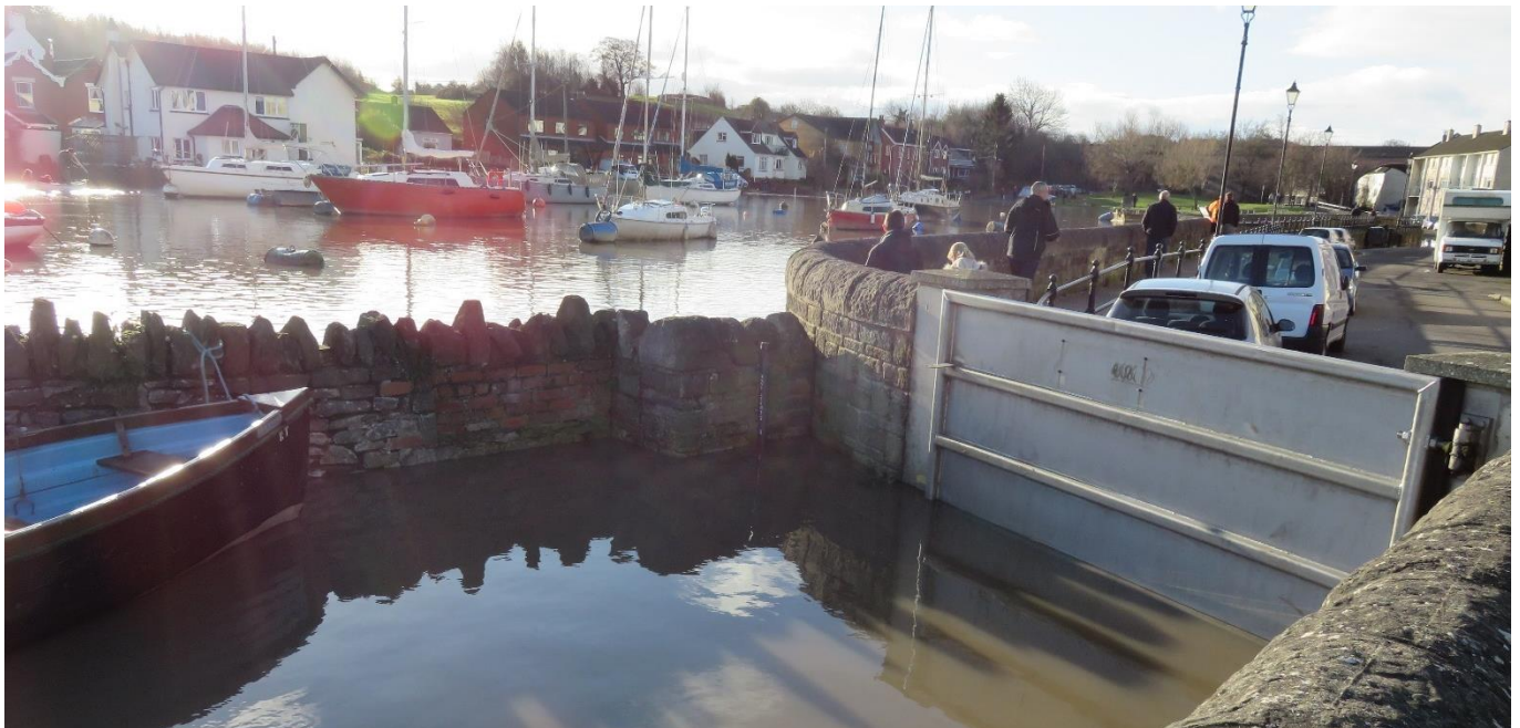
Figure 26: Existing flood defences in operation at Pill
