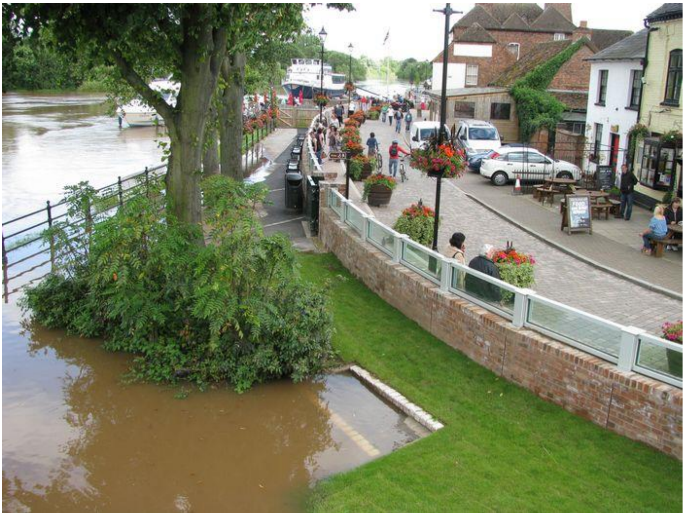
Figure 37: Flood defences including glass panels installed in Upton upon Severn
