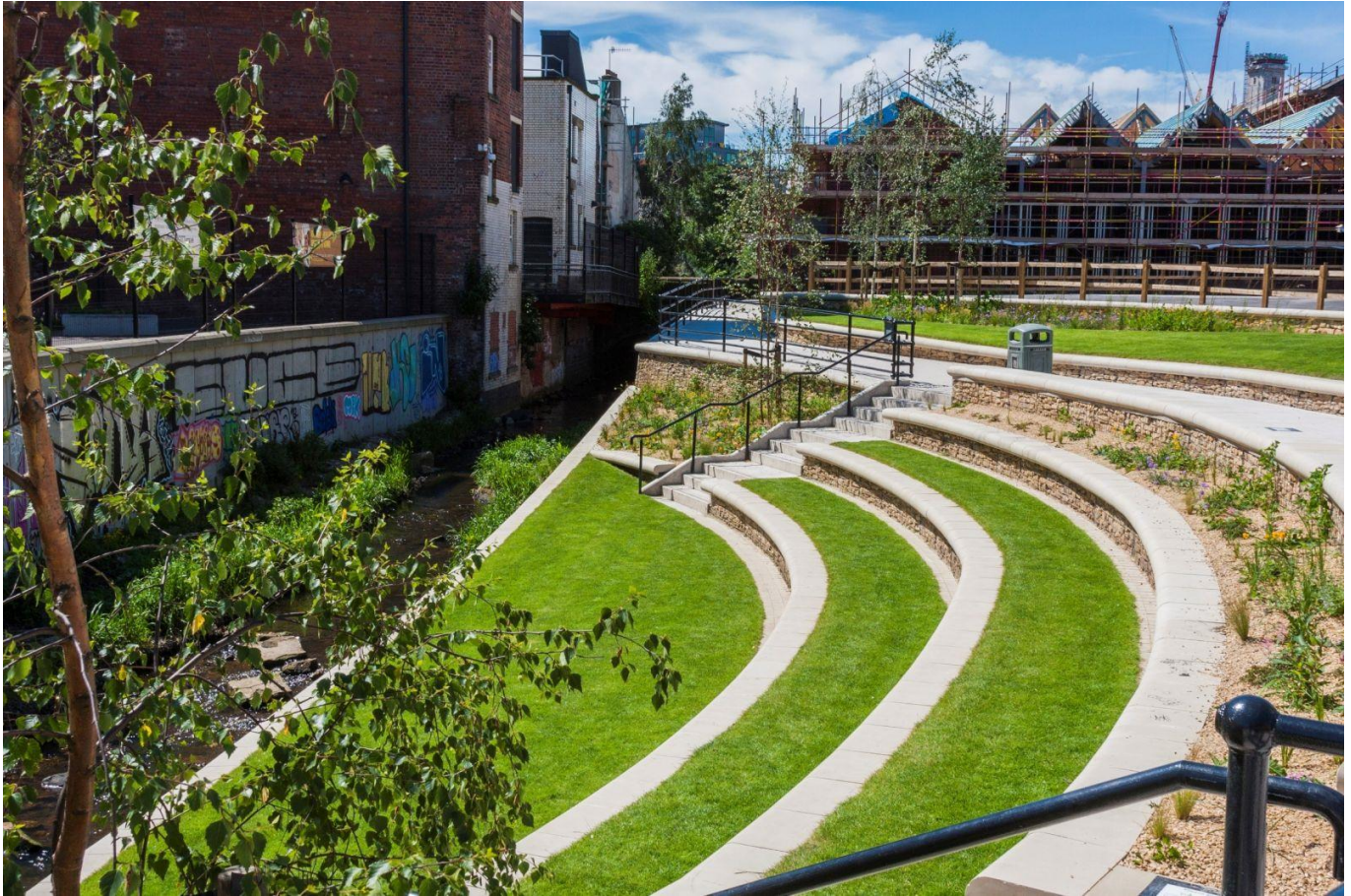
Figure 31: Porter Brook pocket park, Sheffield, winner of the Living Waterways contribution to the built environment category 2016 35
