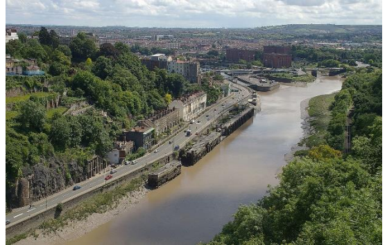
Figure 8 View of Entrance Lock from downstream
