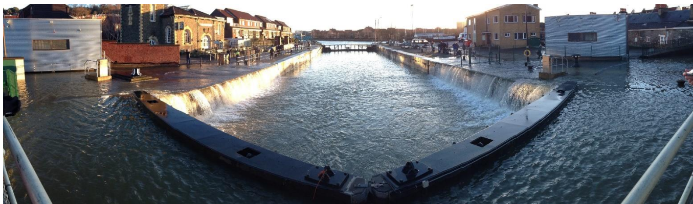
Figure 1: January 2014 tidal surge inundating the A4 Portway in the Avon Gorge (top), Cattlemarket Road (left) and Clarence Road (right), and outflanking tidal flood gates at Junction Lock into the Floating Harbour (bottom).
