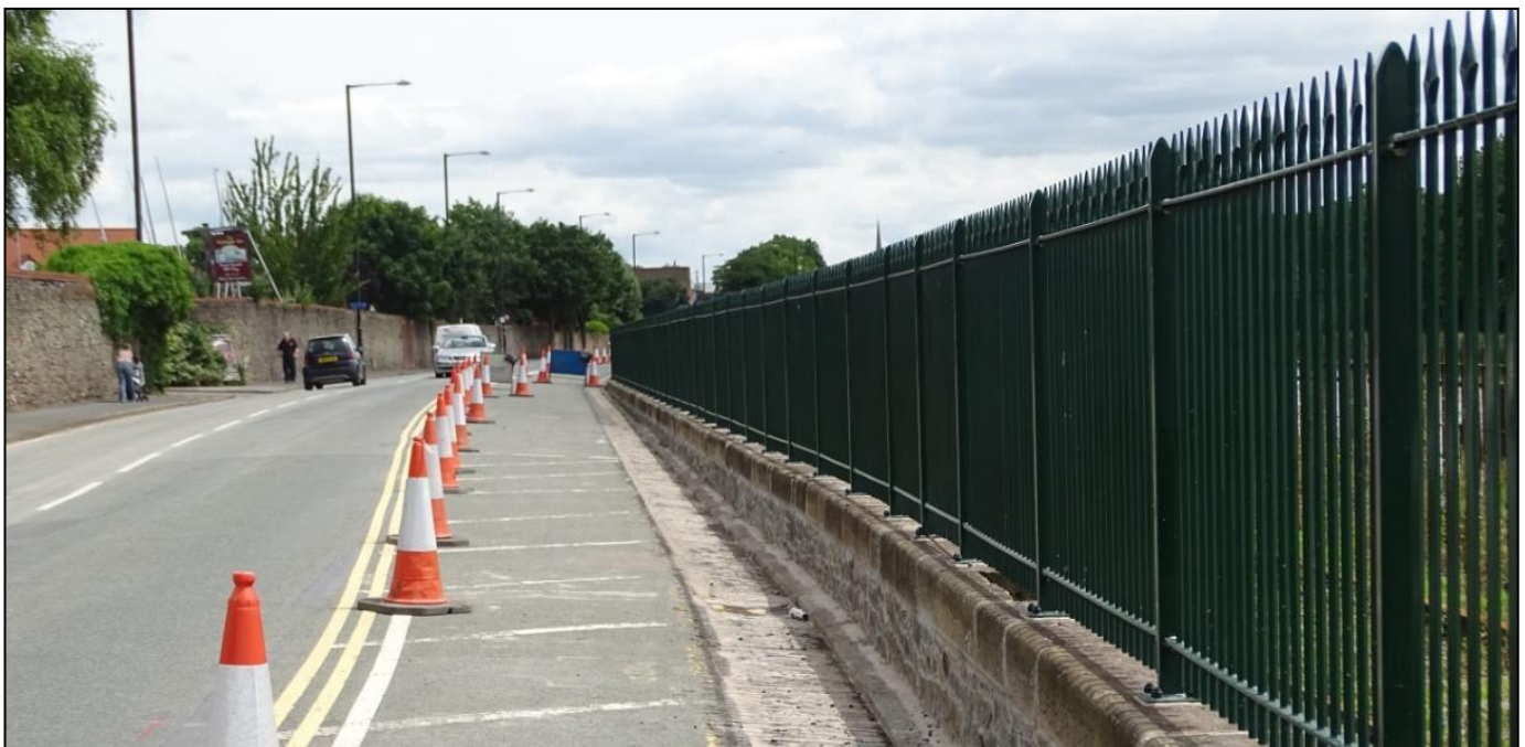
Figure 22: The MetroBus flood wall on Cumberland Road
