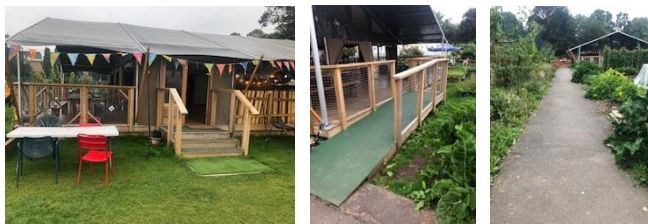
Double steps access with matting and anti slip step covering . Provision of ramp for disabled individuals with path leading from one of the entrances
