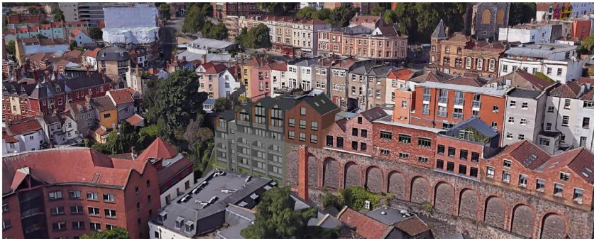
Photomontage 1. Aerial view showing the rear elevation of no. 1A Colston Yard that will be converted to an HMO and the adjoining new-build block containing the serviced apartments.
