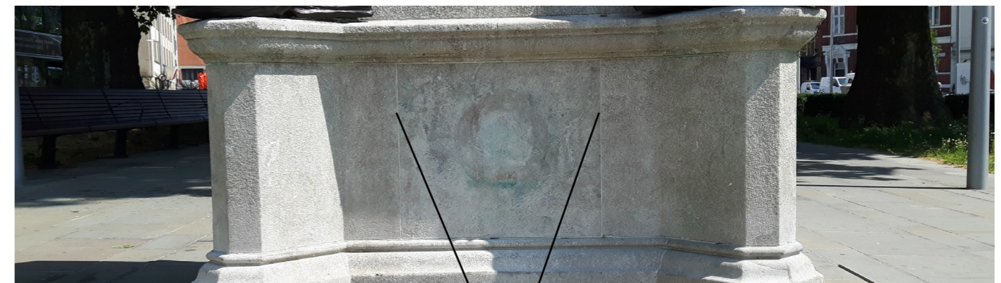
Mortar joints on pedestal
